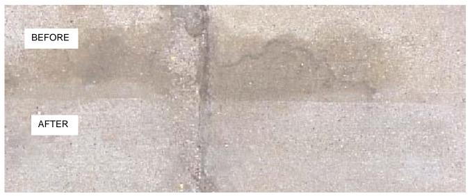
This bottom half of this area was first cleaned with METSO-CLEAN 3755 and then sealed with CONSEAL 1010.
